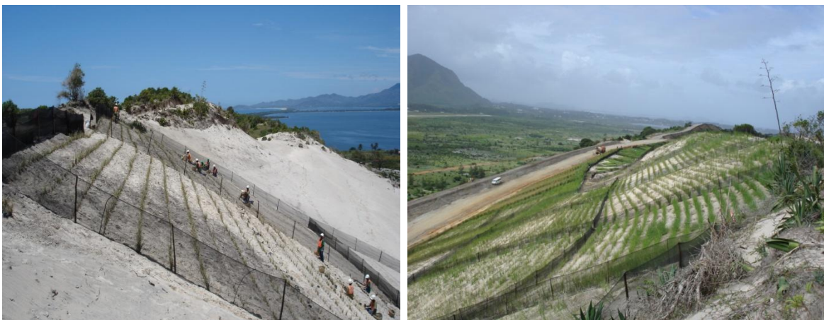
Before and after result of Roley Noffke's work on coastal dune stabilisation
