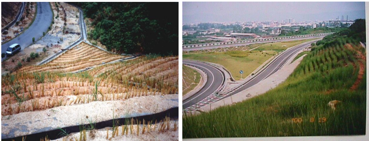
Before and after vetiver planting on a highway in Fujian province
