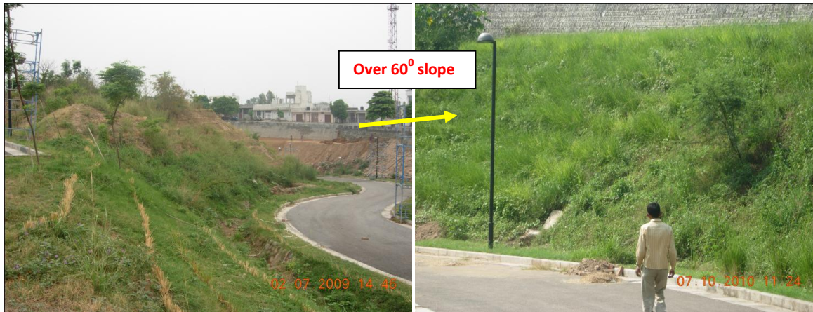
Before and after result of MP Singh erosion control work in Punjab
