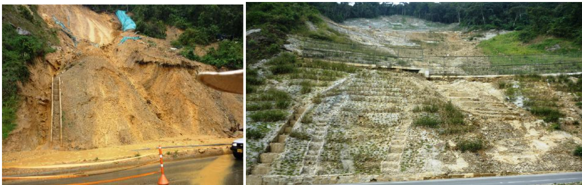
Before and after result of Jorge Lodono's work on landslide stabilisation in Colombia
