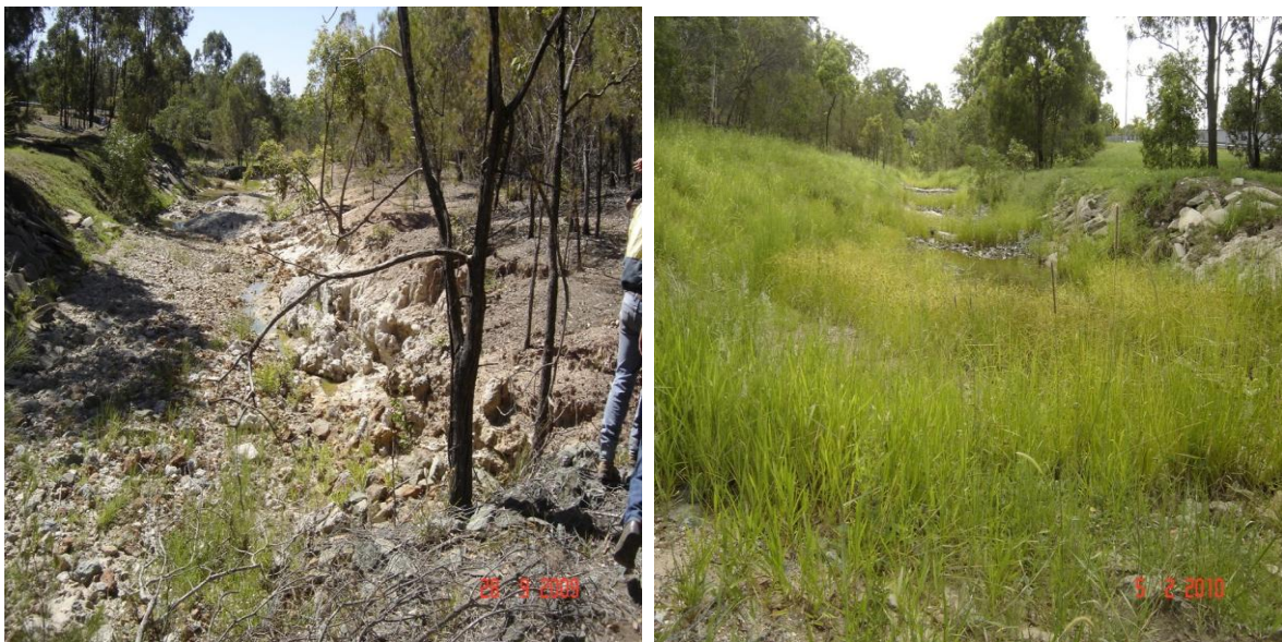
The badly eroded drain before and after vetiver planting. Vetiver conditions before the flood
