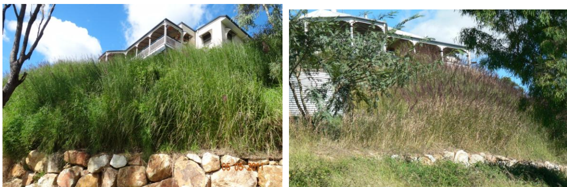
The house was fully protected during the record breaking rain fall in January 2011
