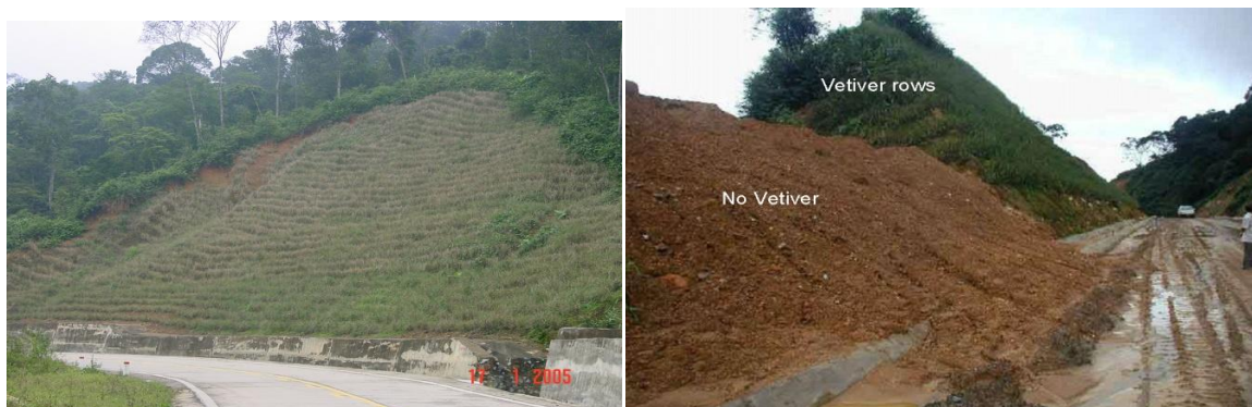
Before and after Vetiver planting on a very steep cut batter of the HCM Highway
