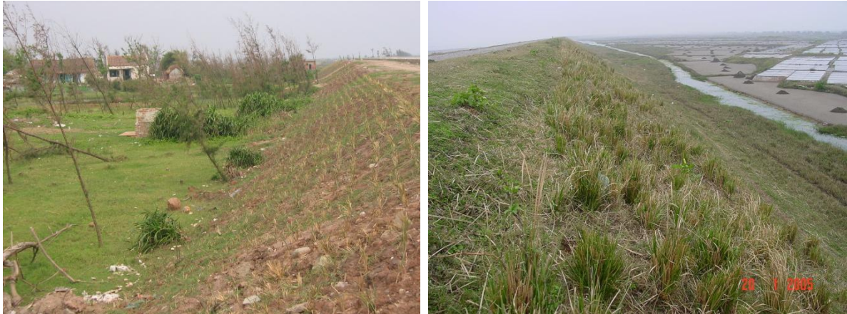
Before and after Vetiver planting on a sea dike in Hai Hau, north Vietnam
