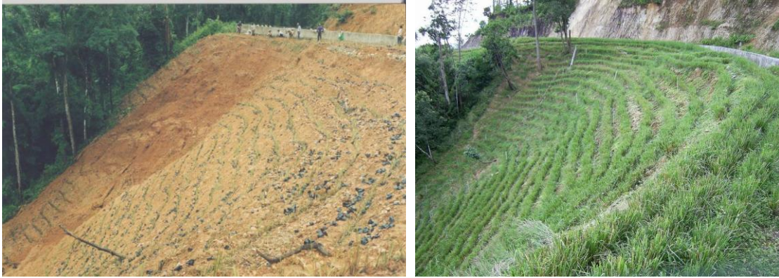
Before and after Vetiver planting on a very steep fill batter of a road in Thailand
