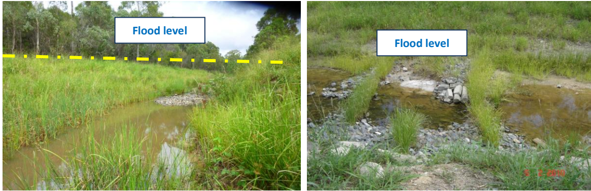
Vetiver planting after the flood and no damages to the banks during flood (left) when flood level almost topping the banks. Flood washed away rock on the groyne while vetiver stayed put (right)
