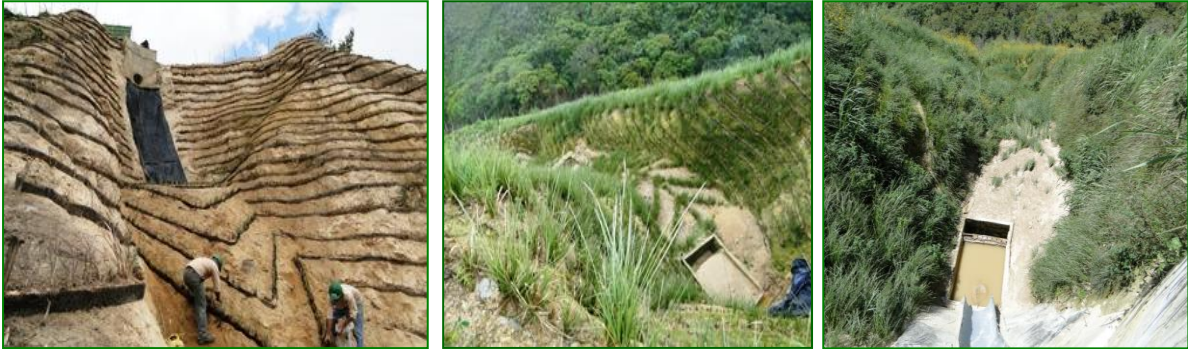
Before and after result of Raphael Luque's work landslide stabilisation in Venezuela
