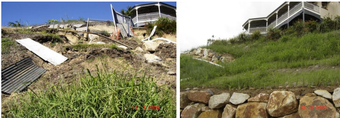
Landslide threatened the foundation of this house on a very steep hill. The slope was repaired and vetiver planting provided full protection two years after planting
