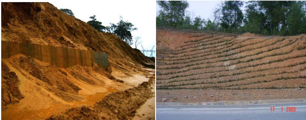
Before and after Vetiver planting on a very steep cut batter of the HCM Highway
